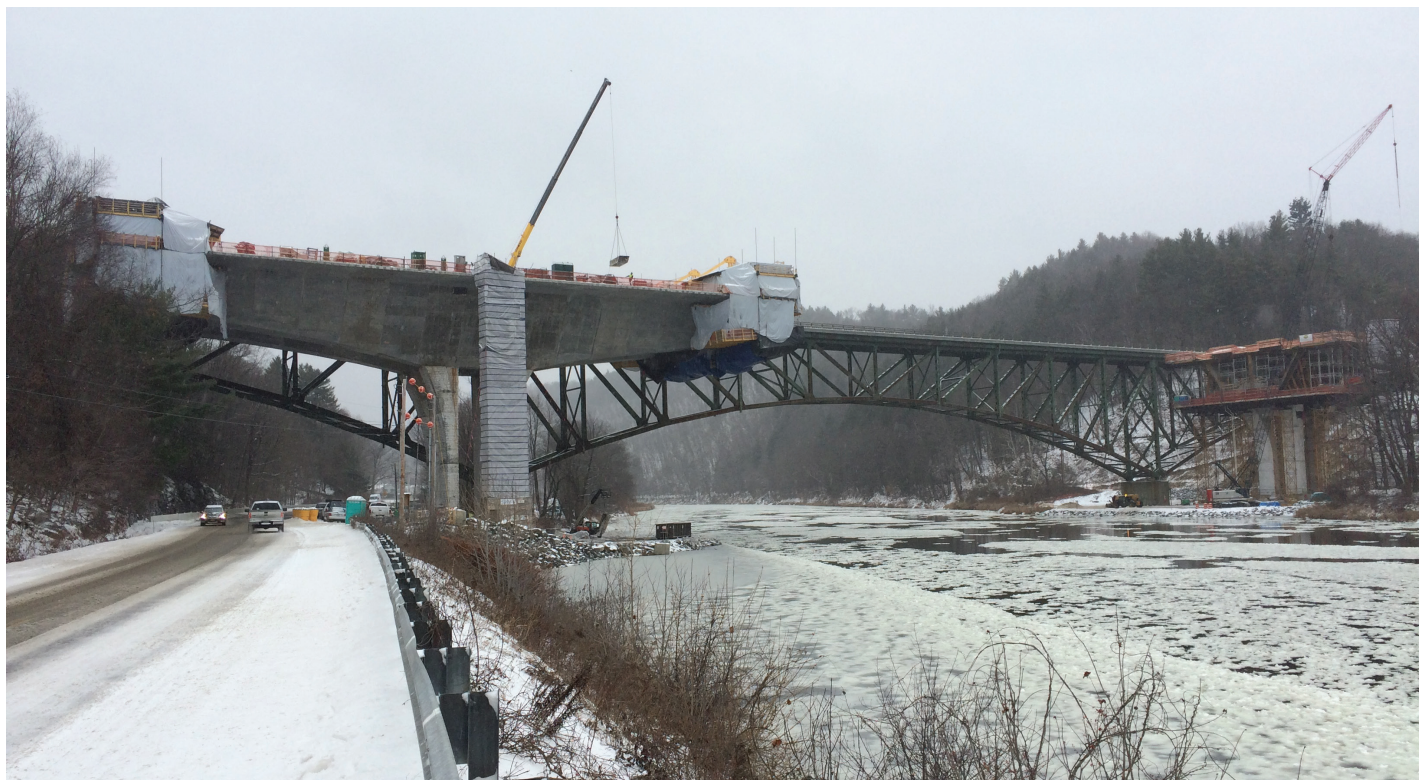
Fig. 2—Construction of the Brattleboro Bridge using segmental concrete balanced cantilever construction.
