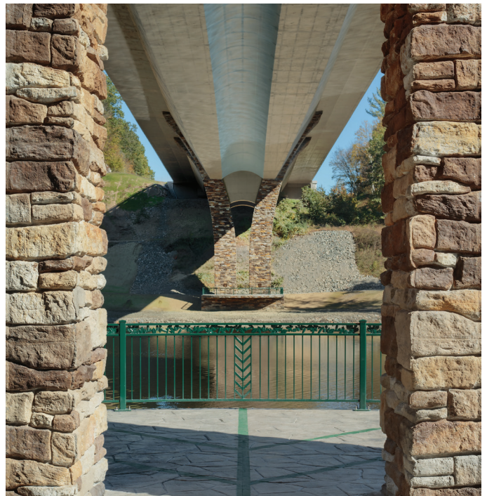
Fig. 5—Stained arch barrel on the bottom of the superstructure.
