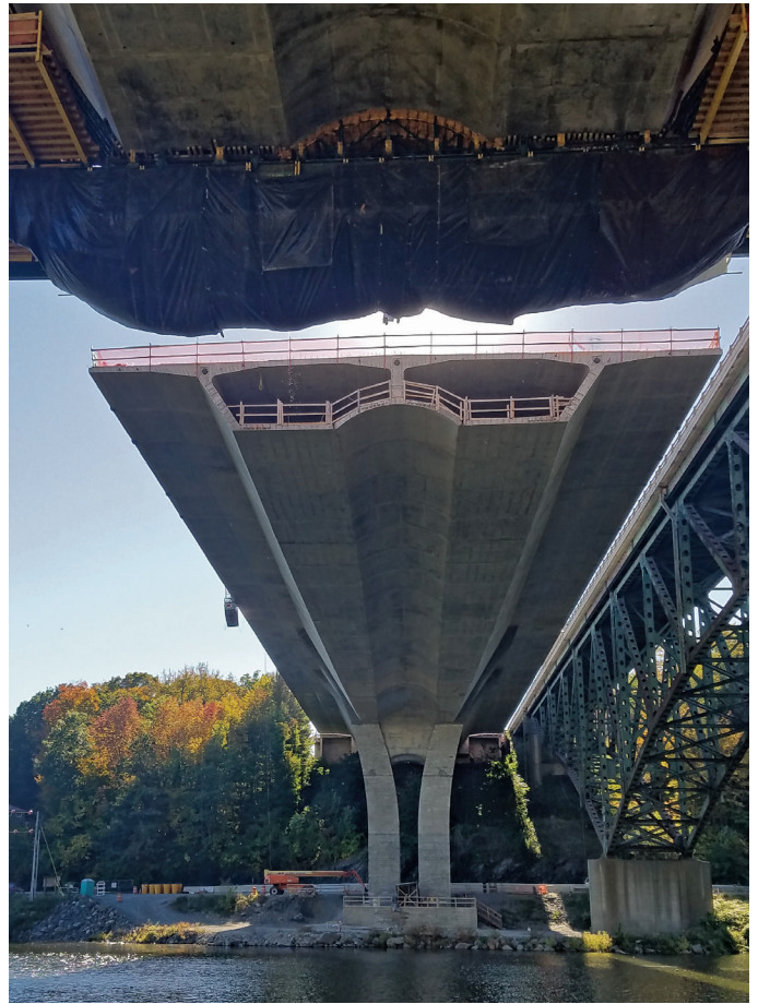
Fig. 4—Trapezoidal box-girder section.
